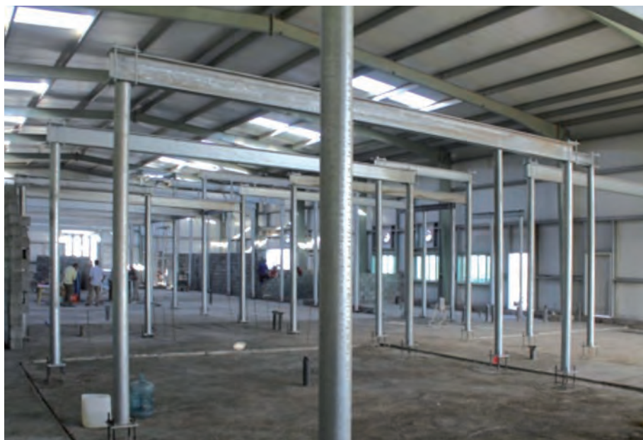
Travi e colonne in acciaio zincato, di sostegno guidovie Rail's supporting structure composed of hot galvanized beams and columns
